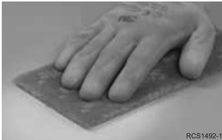
Figure 3. Roughen surface for best adhesion of solar panel
