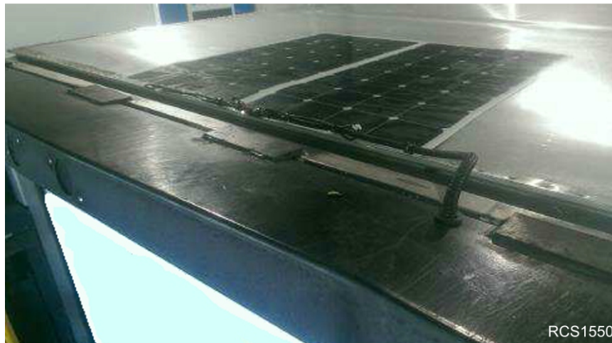
Figure 10. Panels shown installed at rear of trailer.
