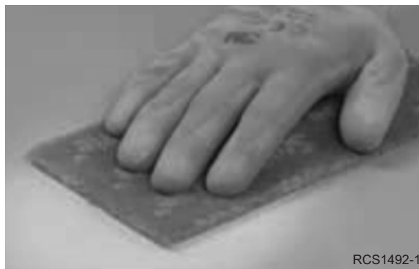
Figure 2. Roughen surface for best adhesion of solar panel
