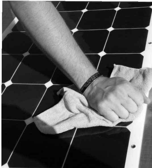
Figure 4. Firmly press panel down over entire area
